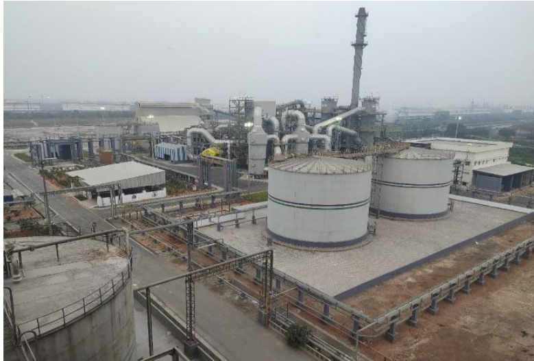
1650 MTPD Sulphuric Acid Plant - III
