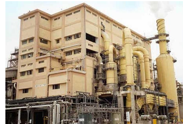
2000 MTPD Complex Plant Train C
