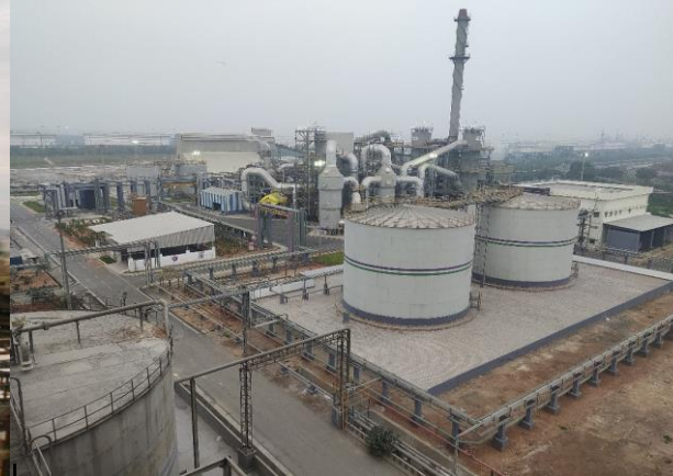
1650 MTPD Sulphuric Acid Plant III
