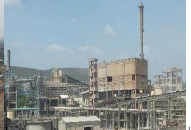
800 MTPD Phosphoric Acid Plant I
